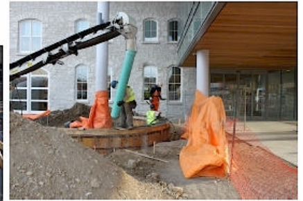
Pumping concrete for benches at City Hall entrance.
