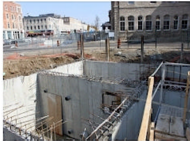
Pavilion foundation walls in place.
