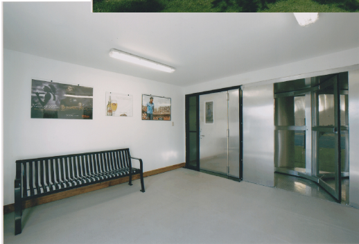
Interior of entry building showing personnel air-lock (for barrier free access) and revolving door into the air-supported structure.
