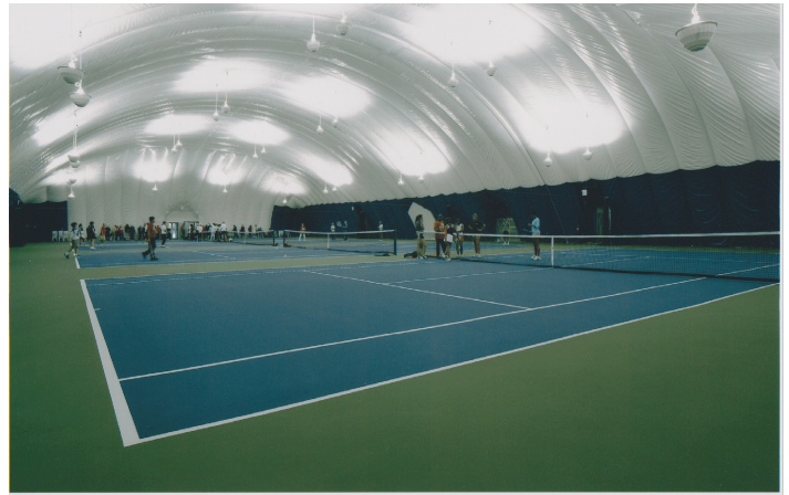
Interior of a new 4-court air-supported structure for the City of Toronto's Tam Heather Curling and Tennis Club.
