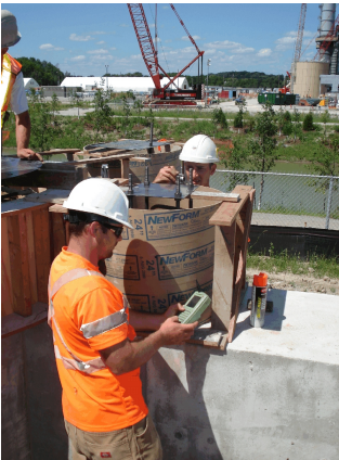
A total of 380 anchor bolts were set. The massive steel structure, along with its complex curvatures required that all field layout be within the strictest of tolerances. The crew from Van Harten Surveying utilized the latest technology in GPS and Total Station survey equipment (see below).
