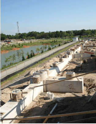
A total of 380 anchor bolts were set. The massive steel structure, along with its complex curvatures required that all field layout be within the strictest of tolerances. The crew from Van Harten Surveying utilized the latest technology in GPS and Total Station survey equipment (see below).
