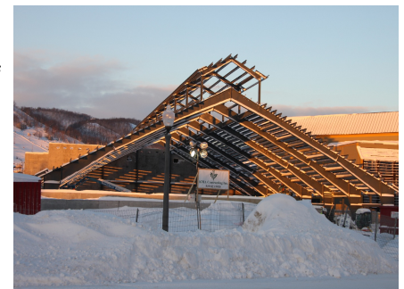
Structural steel framing takes shape.
