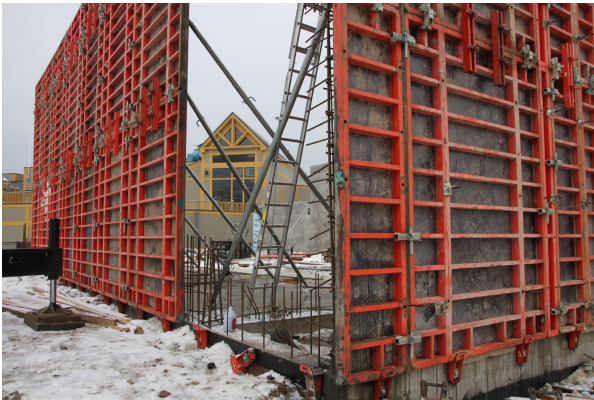
Formwork in place for the 24' high concrete walls.
