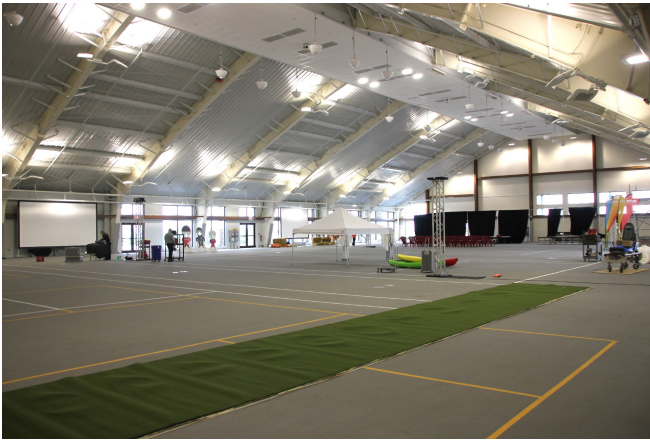
Interior of new conference / tennis hall.
