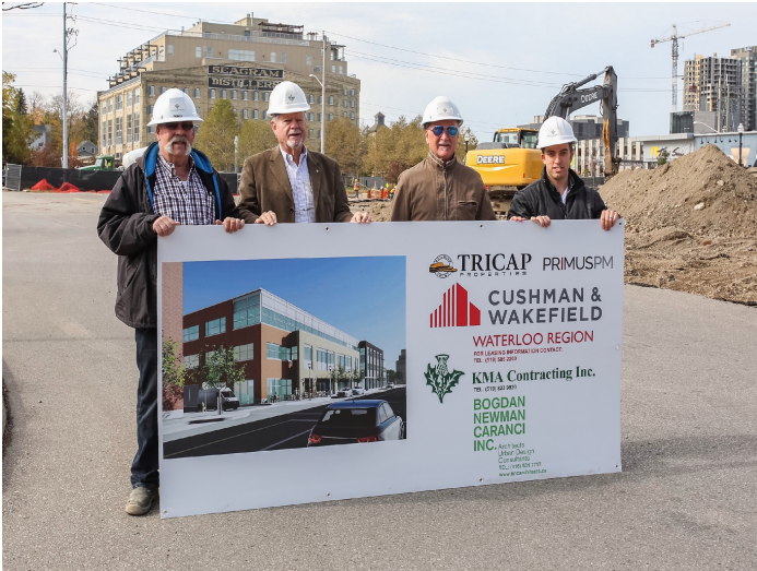
Construction start-up. L to R: KMA's Emmanuel Varem, Superintendent; Keith McEwen, President; Gary Hastings, Project Manager and Nicolas Burt, Project Co-ordinator.
