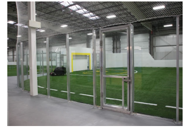
Artificial turf field viewed through a fully glazed dasher board system supplied by The Welmar Group.
