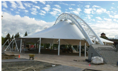
Full pavilion cover in place.
