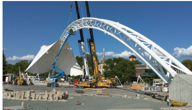
Main support arch complete. Performance stage cover in place.
