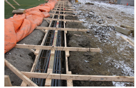
Lakeshore Collegiate's air-supported structure foundation ready for concrete.
